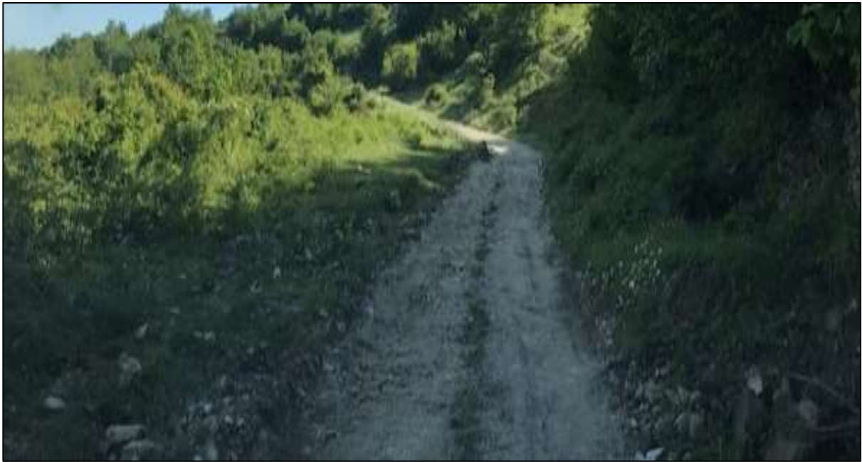
Figure 47: Spoil Disposal Site Access Road
